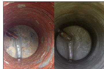
Before (left image) and after (right image) example of Quadex® Qm-1s Restore applied to a vertical shaft originally constructed of brick – image from Vortex technical data sheet
